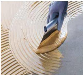
Picture 2. Plank Bonding
